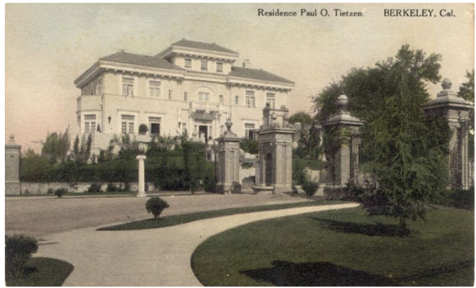
Claremont Court, Berkeley, the Mason-McDuffie development that led to the creation of single-family zoning
